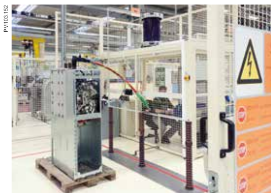
High voltage test
